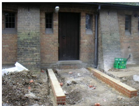
The ramp to the Parish Room door is in progress.
