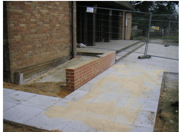
The ramp to the main door is in progress.
